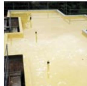
to the substrate underneath. As a result, water cannot flow under the membrane coating, avoiding damage to the roof structure and to furniture and equipment in rooms below.
